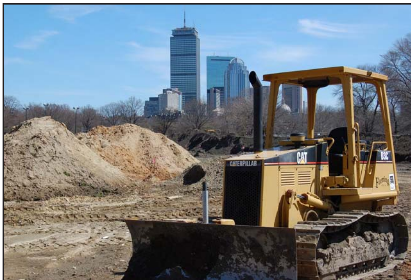
A recent photo of the renovation taking place at Clemente Field.
